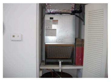
A 710kW heat strip in the air-handling unit provides heat. The heat from the heat strip was recorded at 108°.
